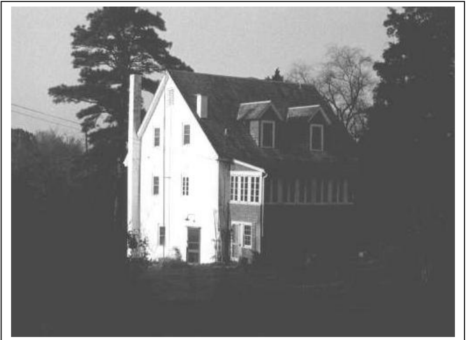
Higgins Mill, 1976 photo by Michael Bourne for MHT
